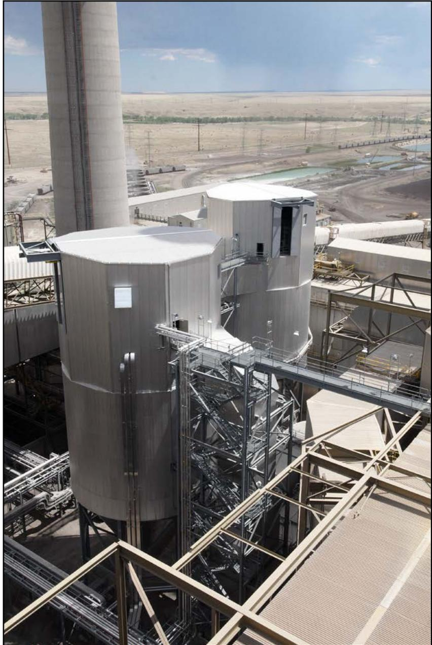
*The unique flue gas dispersion system, coupled with the reliable atomizer, allows optimal gas and reagent mixing for high SO<sub>2</sub> removal efficiencies.*
