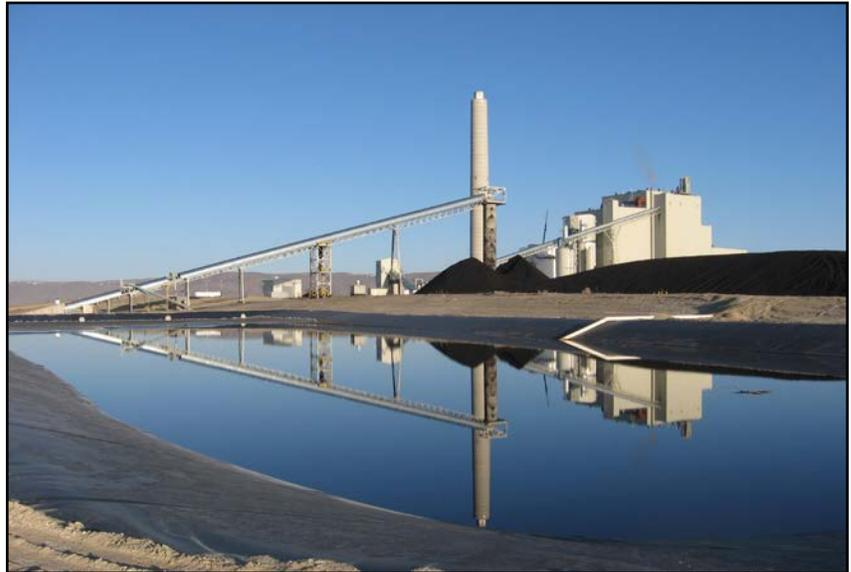
*The Newmont Mining TS Power Plant, featuring a B&W RB Carolina-type pulverized coal-fired boiler, will supply electricity to Newmont Mining Corporation's operations in northern Nevada.*
